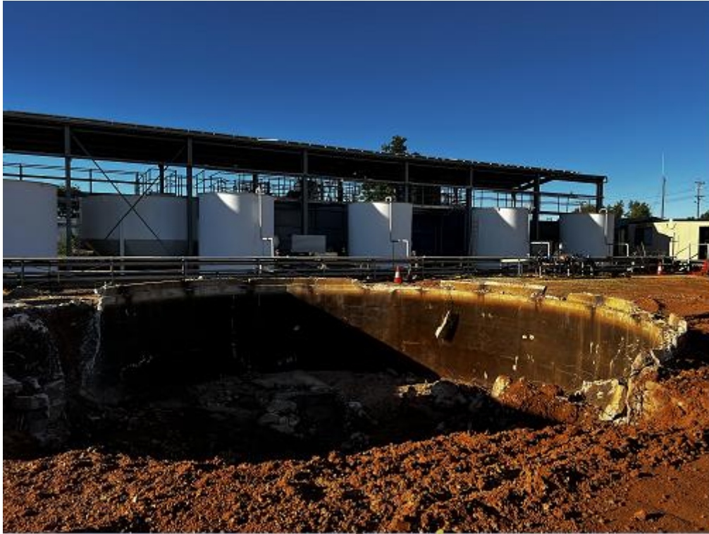
Photo 2 – Reservoir Demolition WTP
