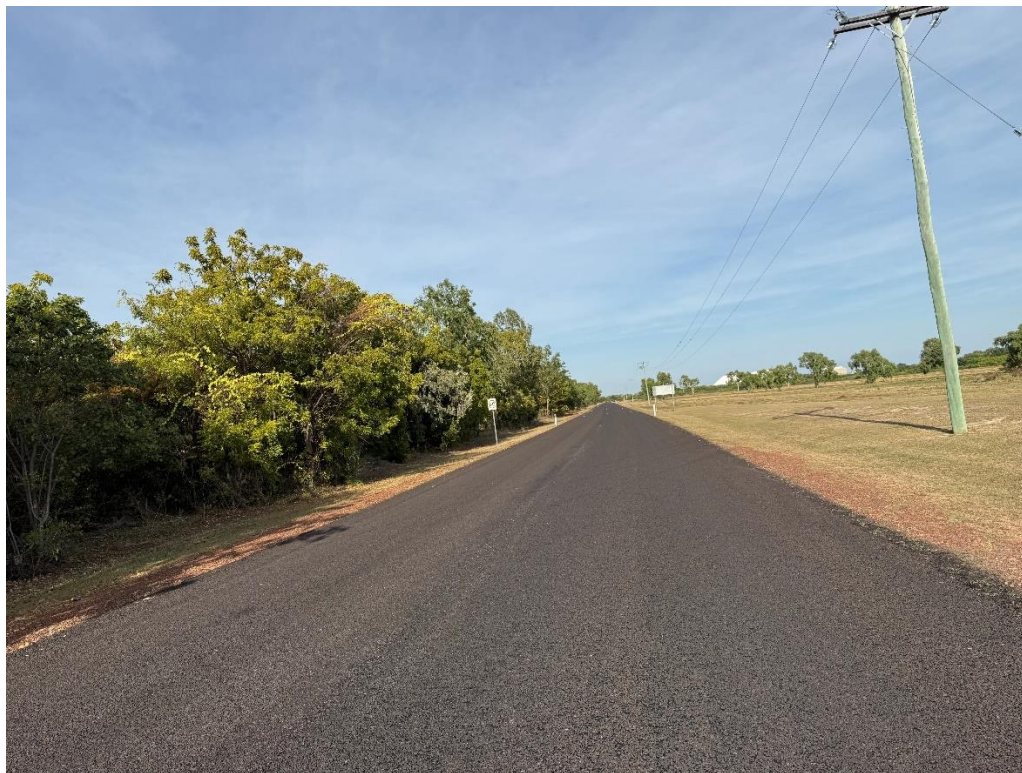
Photo: New 10mm reseal – Truck Bypass Road Karumba
