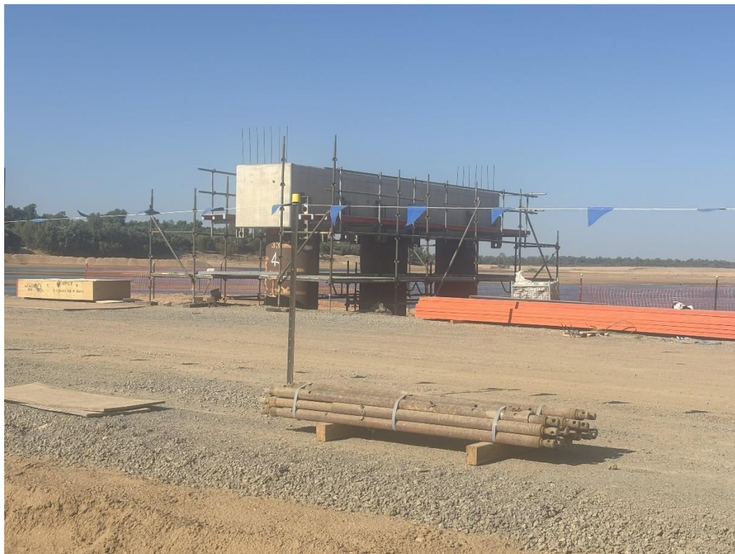
Photo: Mitchell River Placement of headstock
