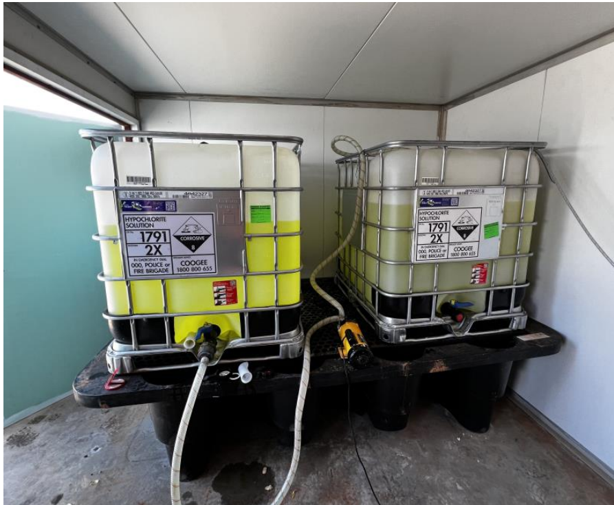
Photo 3 – Chlorine shed internal
