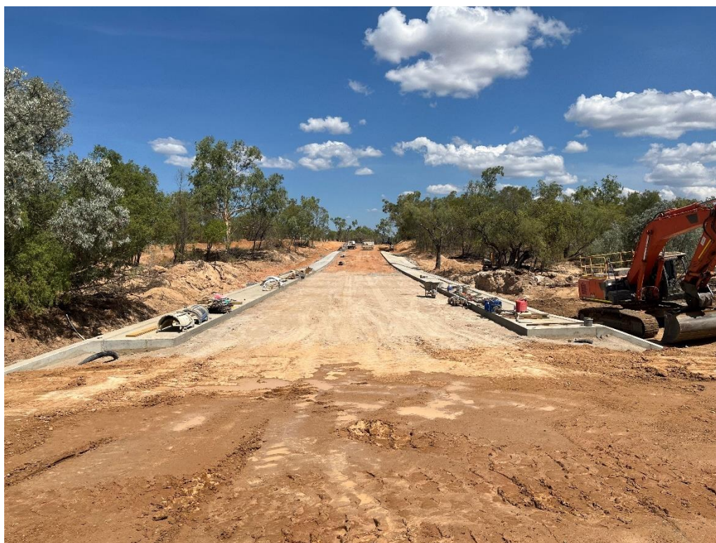
Photo: Clark Creek – Working on the concrete batter protection
