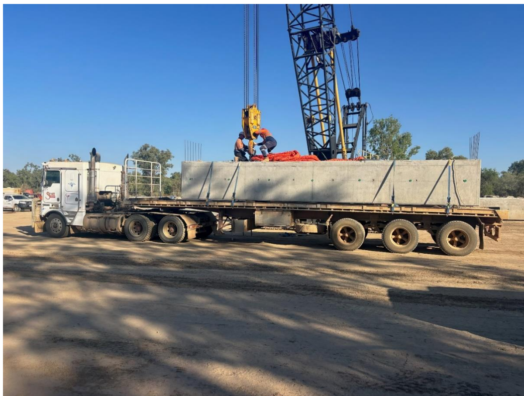
Photo: Mitchell River – Loading the headstock to the top of the steel piles
