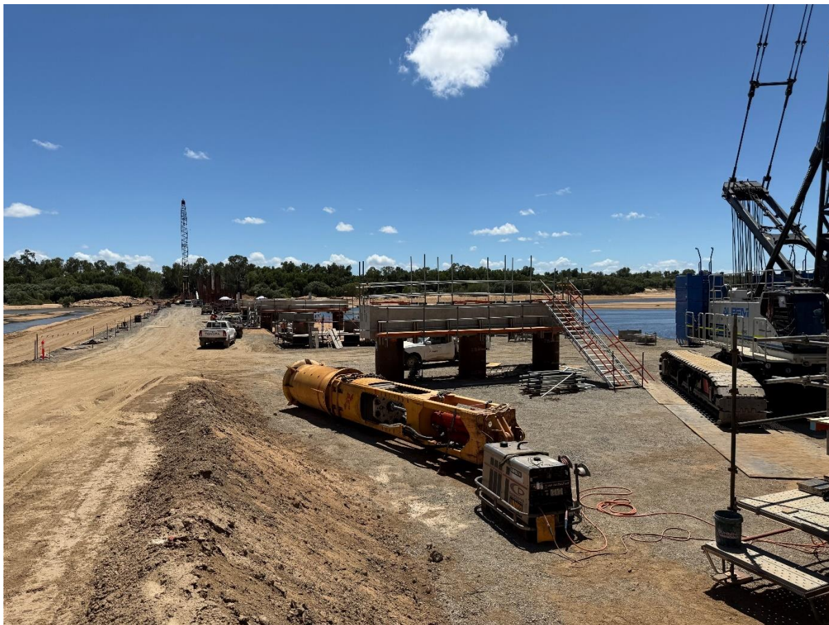
Photo: Mitchell River Placement of headstock
