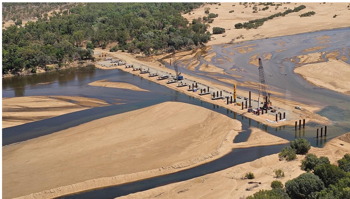
Photo: Mitchell River – seven headstocks installed
