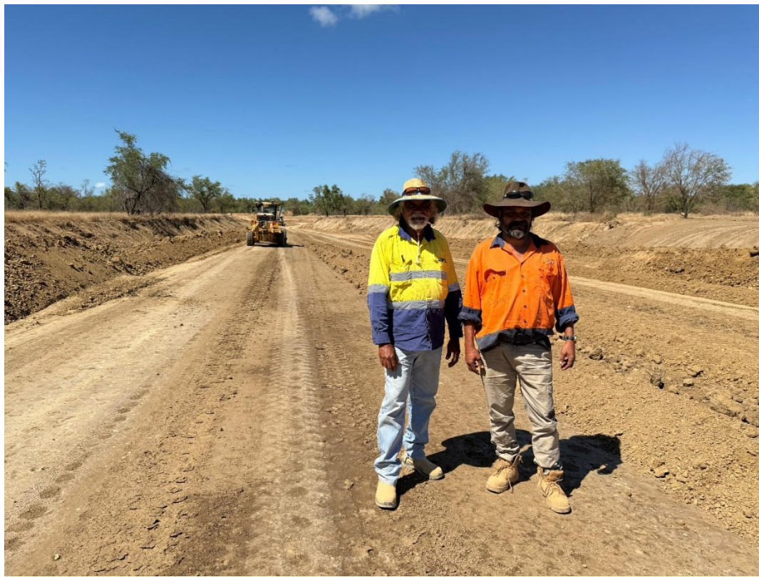
Photo: Koolatah Road – repairing washout.
