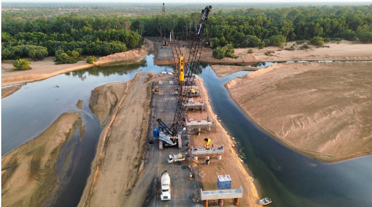
Photo: Mitchell River Placement of headstock – piling nearing completion at north end.
