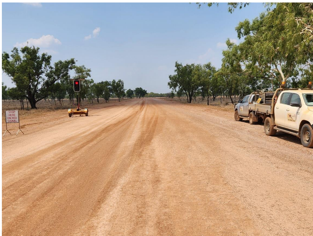
Photo: 89B Betterment 2 – 5.1km of stabilised pavement ready for sealing
