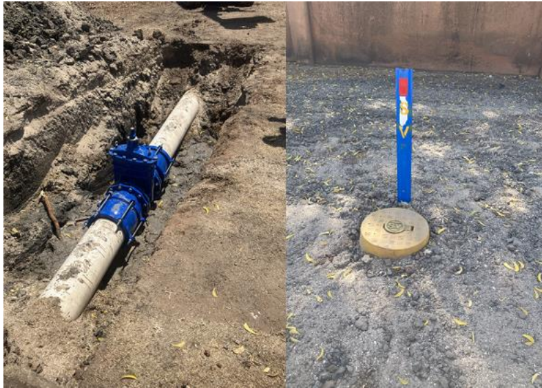
Image1 – New 300mm Valve Yappar Street (before/after)
