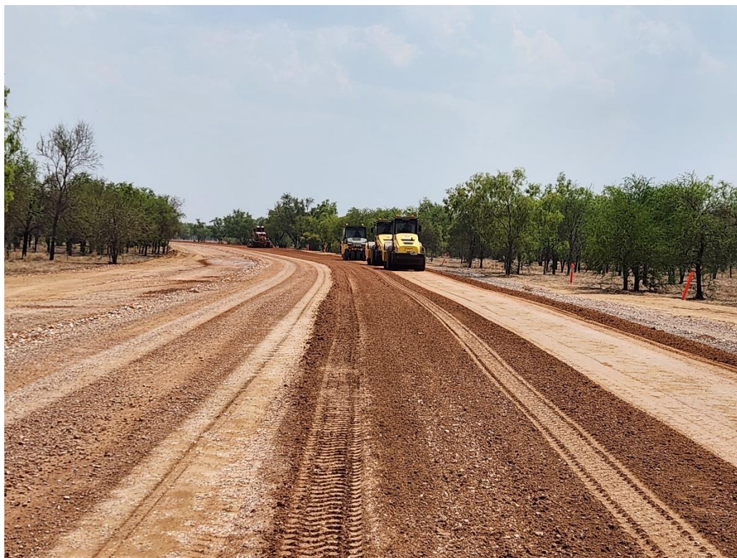
Photo: 89B Betterment 2 Compacting pavement
