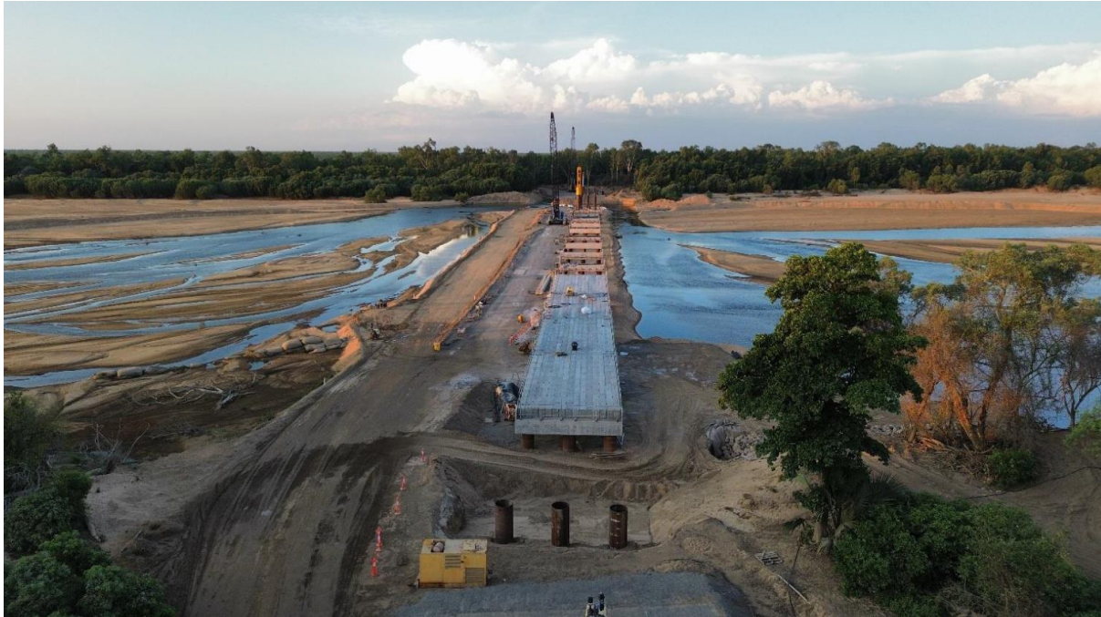
Photo: Mitchell River – 60m of deck installed
