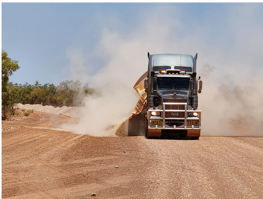
Photo: ROSI Burketown Road – carting gravel
