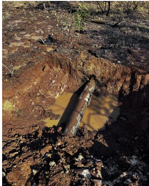
Image 2 – Leak Repair Glenore Raw Water Main
