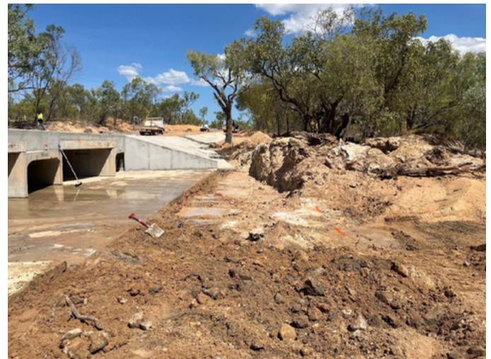
Forming up headwall and batters at Clark Creek
