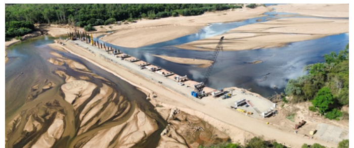
Two headstocks installed
